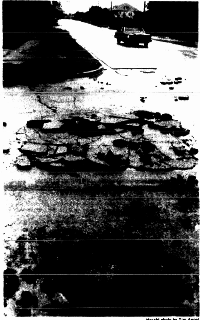
Heavy and prolonged rain this week has created temporary streams rushing through city streets, causing extensive pavement damage in many areas of town. This cracked and crumbled surface is at the intersection of Eighth and Scurry streets.
