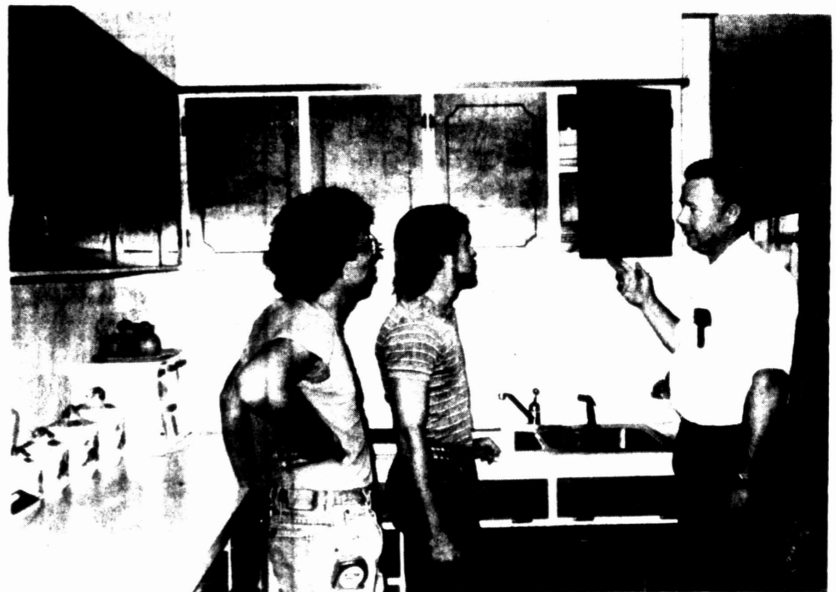
CABINETS — Rod Zapata, Craig Neighbors and Bob Noyes look over cabinets they recently built and installed in a Kentwood home.
