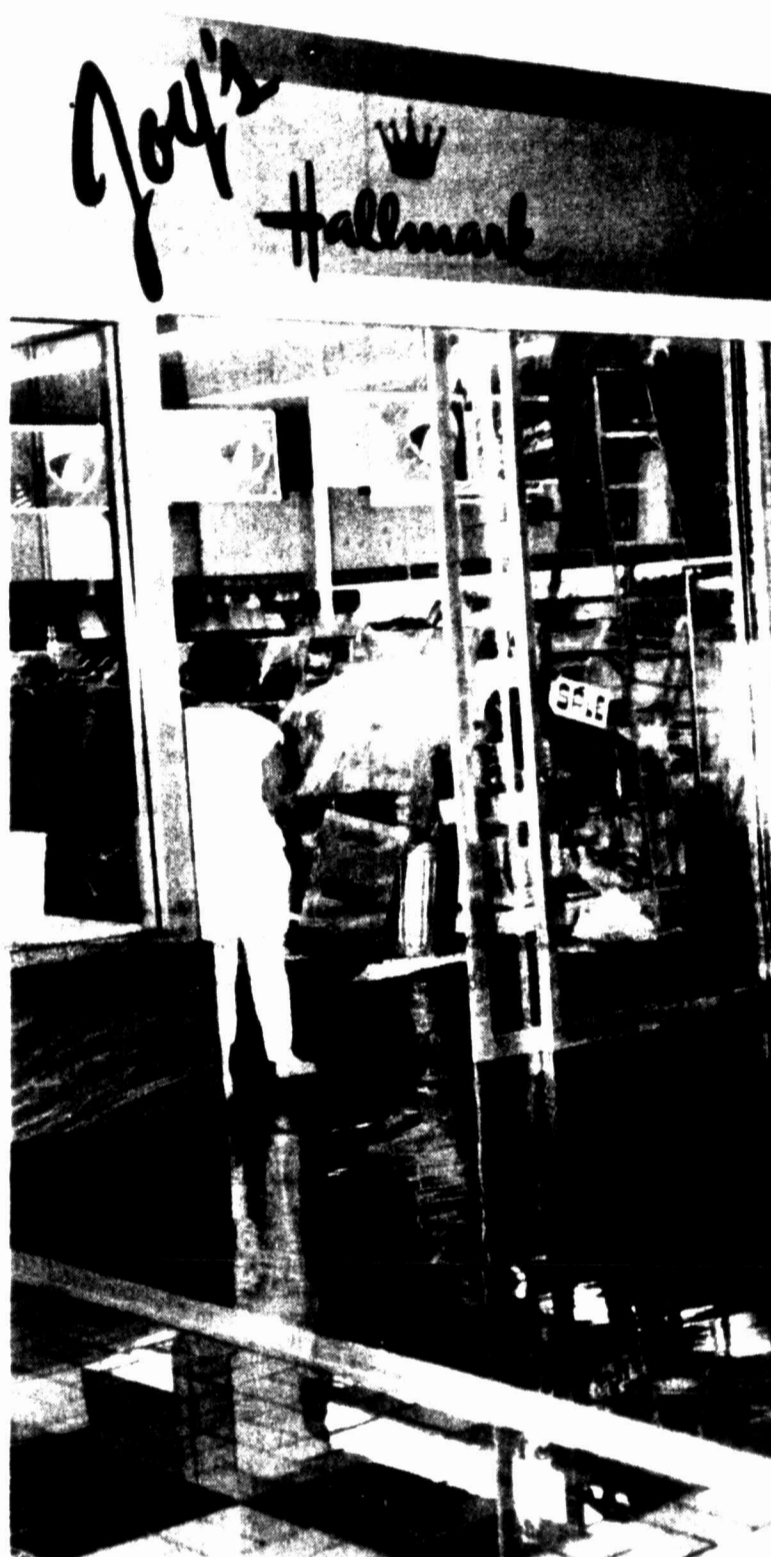
Water pours through the ceiling of Highland South Shopping Center Saturday, the result of a clogged drain. The shopping center's walkway flooded, and items in Joy's Hallmark Card Shop were damaged, causing the store to close early.
