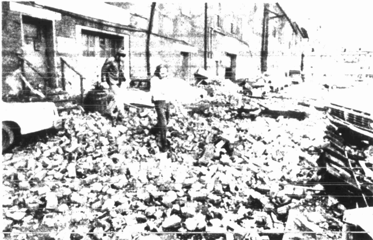
Gary Rhoton and Lee Rickett walk across a street littered with bricks from a fallen building damaged by a severe thunderstorm that hit Covington, Ky., late Monday afternoon. Rickett was inside the five-story building when the storm hit and escaped unharmed after digging himself out.
