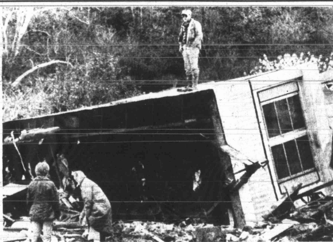
Many residents were still looking for their homes Wednesday after record flooding washed them away. This family was luckier than some and found their trailer home washed down the road a short distance.
