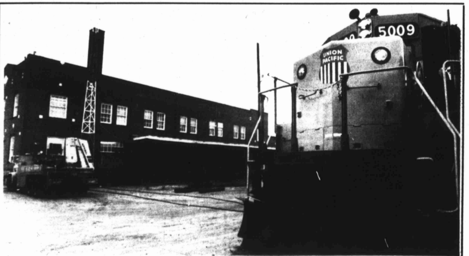
Missouri-Pacific freight depot in Big Spring is scheduled for destruction.
