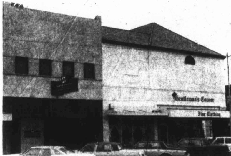
A DIFFERENT LOOK — Above is the Staked Plains Masonic Temple as it looks today. During its remodeling many years ago, the Temple's upper facade was removed. The Temple may be entered at two entrances on the ground floor facing Main Street.
