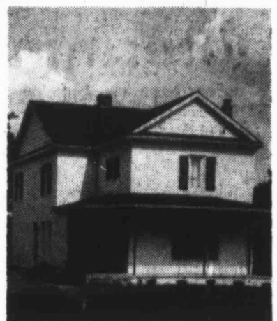
SIDING — Eight-inch panels cover the gables while steel siding panels cover the body of the house, giving a symmetrical look to a large home.
