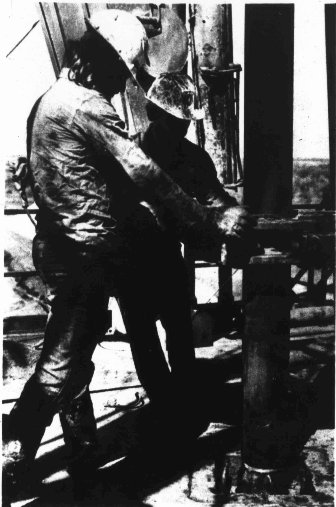
ROUGH WORK — These two roughnecks are getting ready to run in the first piece of pipe to start drilling a well. The pipe, called a collar, is being held by a pair of tongs. The drill bit is attached to the bottom of the collar.
