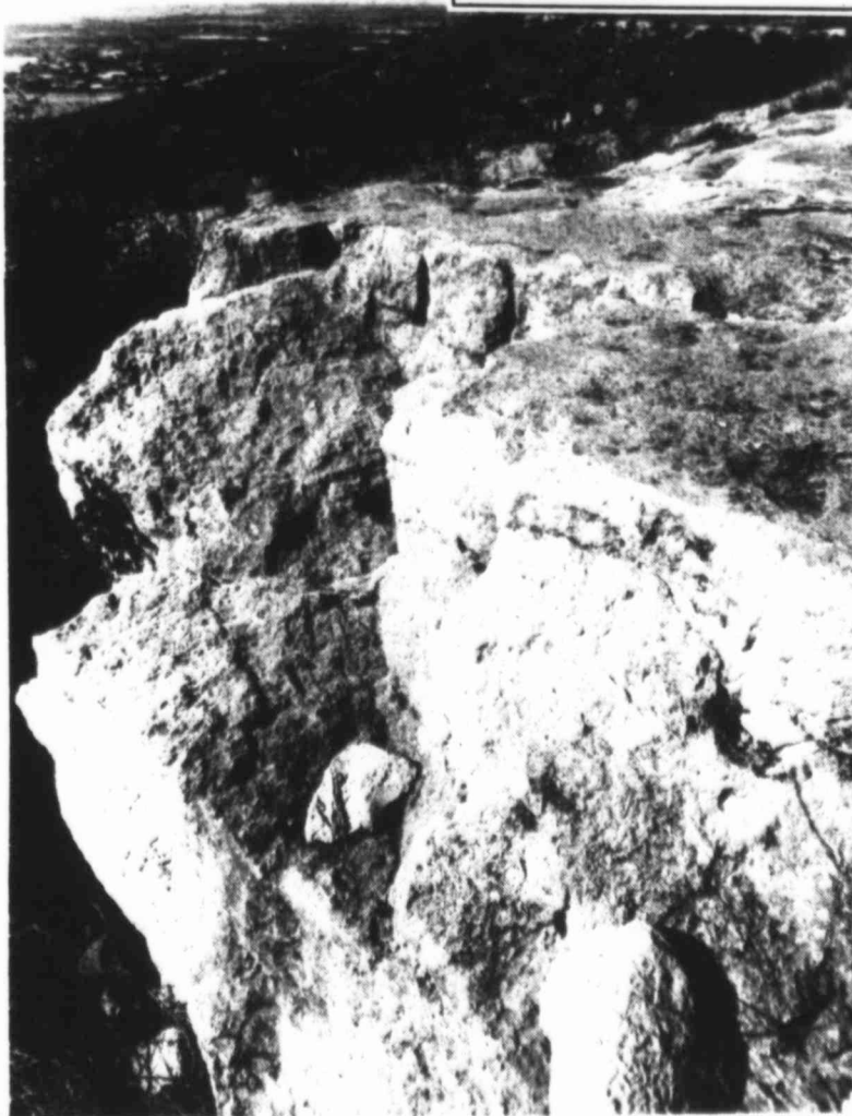
MARKED MOUNTAIN — CCC troops wedged limestone from this quarry on the Western rim of Scenic Mountain to build structures for Big Spring State Park. Wedge marks are clearly visible in the rock.
