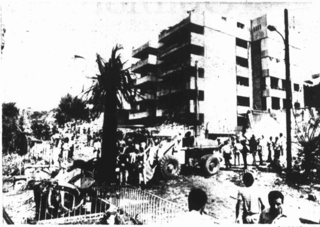
OVERVIEW — A wide shot of the U.S. Embassy annex in Christian East Beirut after a car-bomb exploded here Thursday. More than 20 people were killed and up to 60 were injured in the early-morning blast.
