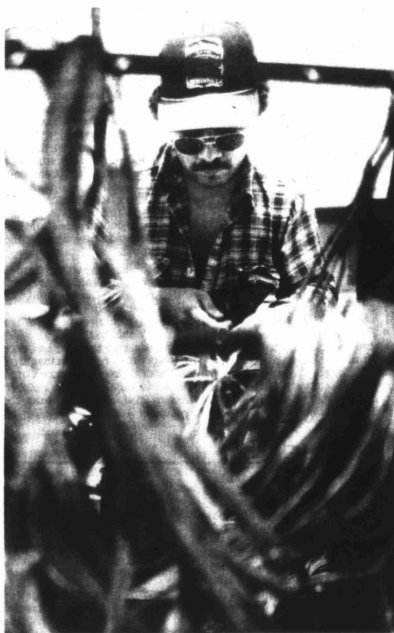
LIVE WIRE — Jimmy Carrillo, an employee for Southwestern Bell, seems to have everything under control, despite the staggering number of wires in the foreground. Carrillo was doing some line work for Southwestern Bell Friday afternoon on Eighth Street.
