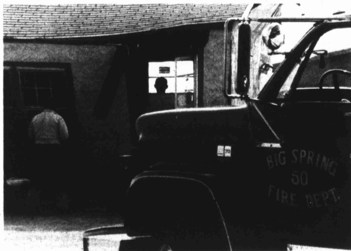
EXPLOSION INJURES ONE — Two Big Spring firemen look over damage caused by an explosion at the Chief Apartments on West Highway 80 about 5:30 p.m. Tuesday. Adolfo Salazar, 37, received second and third degree burns in the blaze, which may
