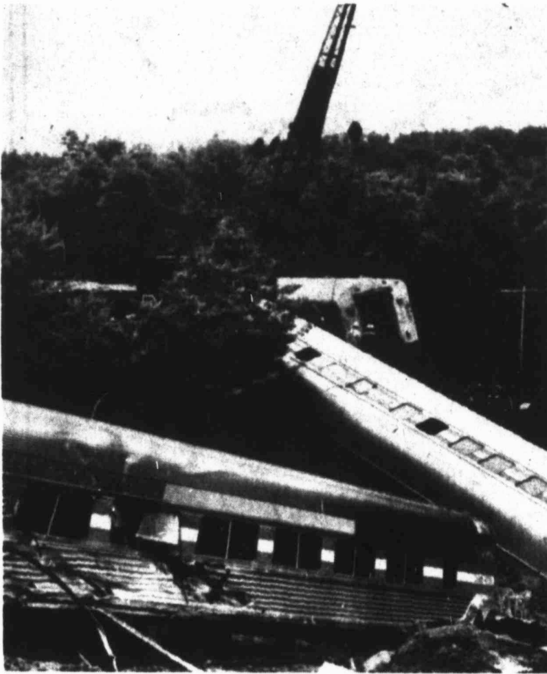
DERAILMENT CLEAN-UP — Amtrak railway cars lay strewn about in Williston, Vt., Sunday as workers using a large crane continue to clear the area in the aftermath of Saturday's derailment which killed five people and injured more than 130 others.
