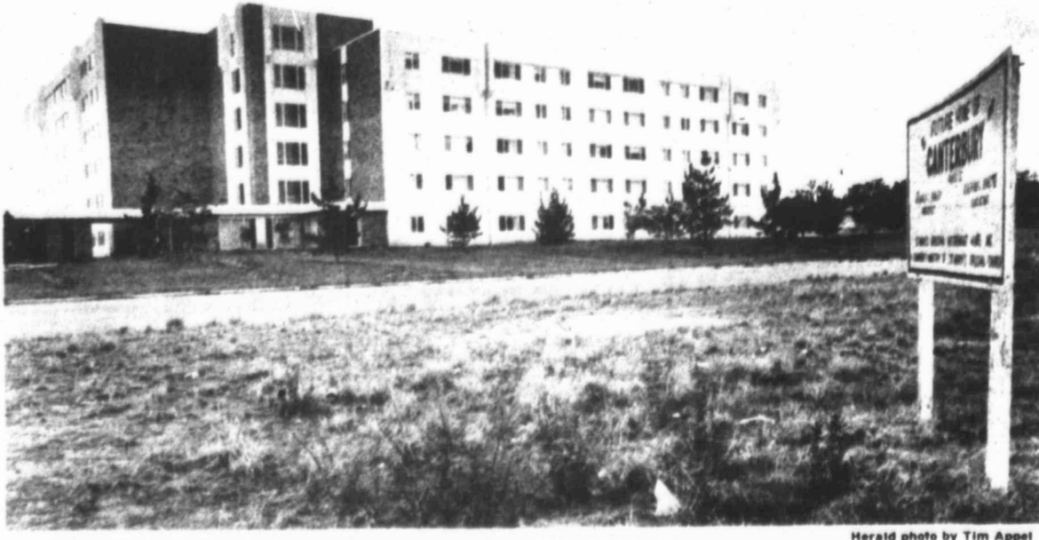
CONSTRUCTION TO BEGIN — Construction on 59 new apartments at Canterbury retirement center will begin next week. Construction had been delayed
