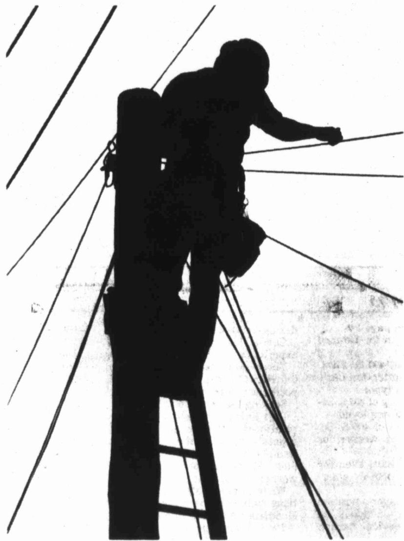
SPIDERMAN — Buddy Miller, an exchange technician for Southwestern Bell, appears to be weaving himself a web as he works on some lines in the late afternoon sun Thursday on Seventh Street between Gregg and Scurry.
