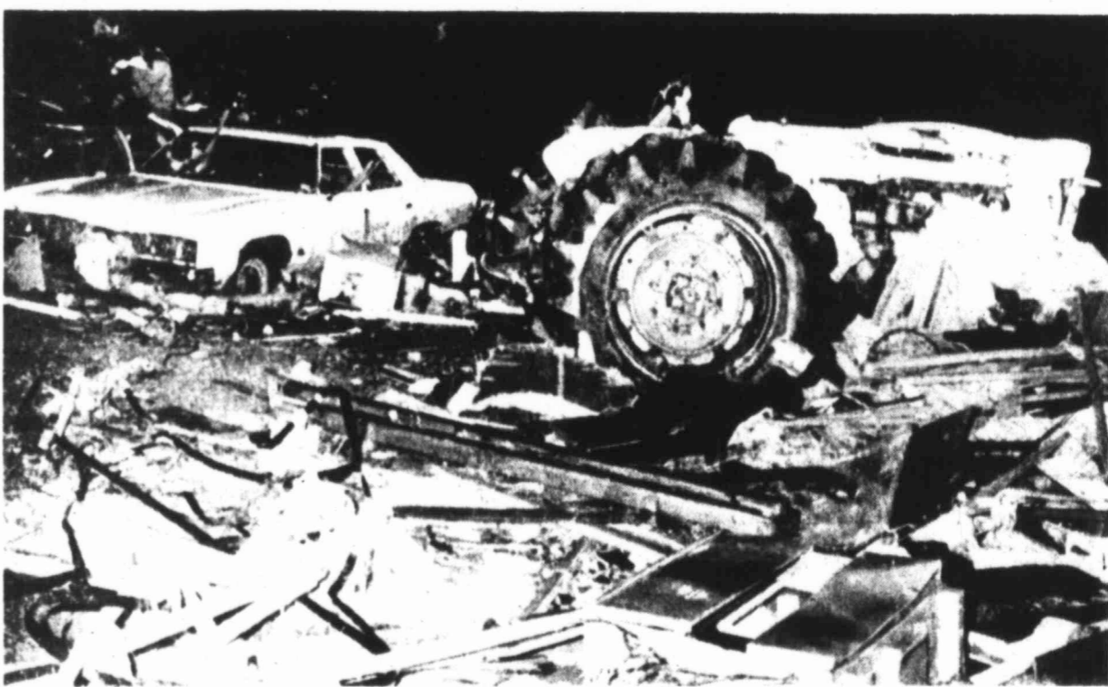
TORNADO DAMAGE — Wreckage litters the town of Fisher, Ark., Thursday night after a tornado ripped through the area, killing three persons. Associated Press photo
