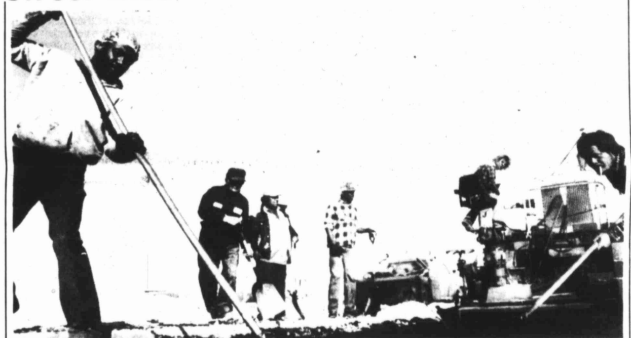
AT LONG LAST — Workers from Price Construction Inc. lay the first asphalt on Birdwell Lane near Sixth Street. Paving on all four lanes of the street from
