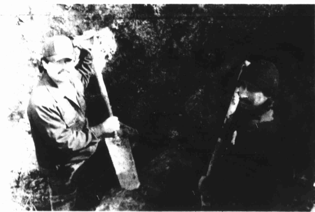
DOWN IN THE HOLE — City utility workers Eliseo Gamboa and Joe Torres dig out around a water main in extreme south Big Spring. Conditions much
