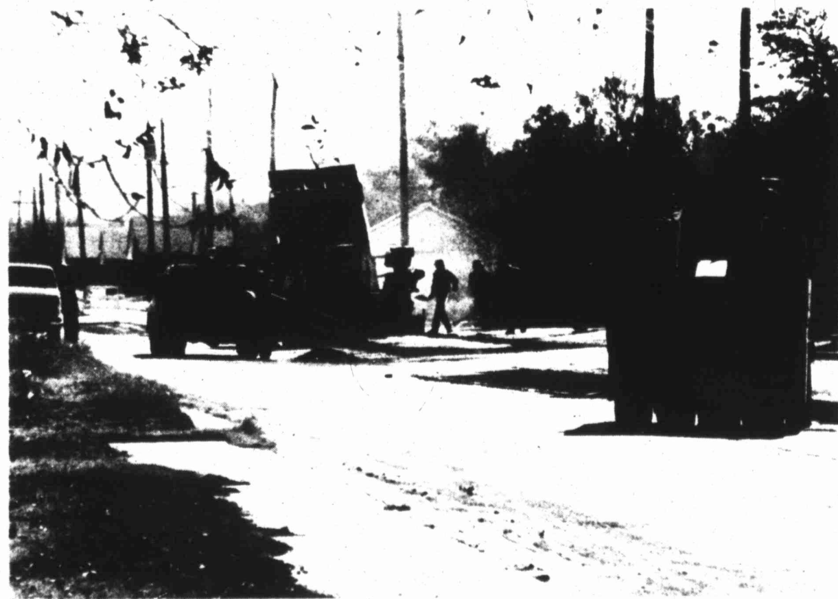
STREET WISE — Price Construction Co. crews lay asphalt Friday on a four-block stretch of Goliad Street which was opened again to traffic late Friday afternoon.
