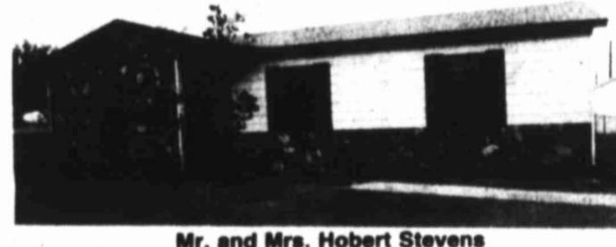
Mr. and Mrs. Hobert Stevens Jonesboro Road Steel siding was installed on entire home, with Coronado rock trim and solid glass storm windows and doors
