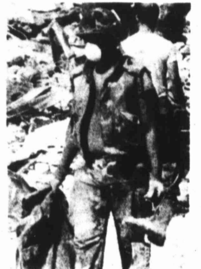
CLEANUP — A U.S. Marine carries boots and a flak jacket from the rubble of their command building this morning. The building was destroyed by a terrorist bomb early Sunday morning, killing more than 140 Marines.
