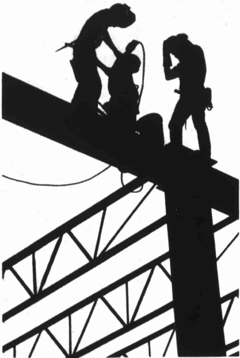
HIGH ON THE JOB — Construction workers in San Antonio are silhouetted against the sky as they go about their duties recently. The workers are welding an office building near downtown San Antonio which will house Control Data Corp., a facility expected to provide 1,000 jobs. Associated Press photo
