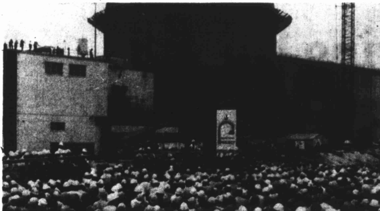
HARD HATS HONORED — More than 4,000 craftsmen and workers were honored Wednesday for their work in completing the first dome reactor building at the mammoth South Texas Project two months ahead of schedule.
