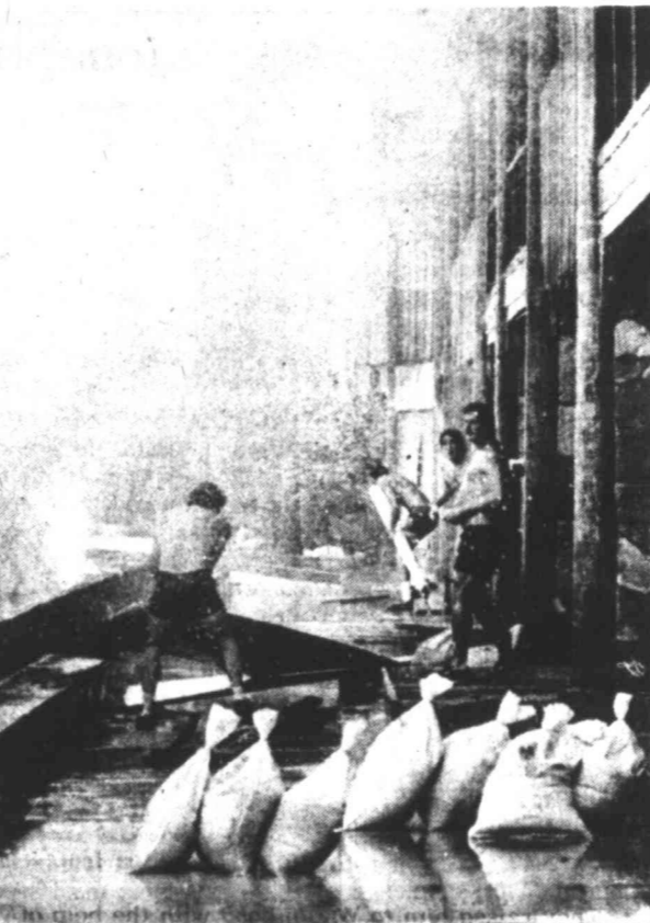
HIGH SURF — Construction crews board up 16 units damaged by pounding surf Tuesday night at Blue Lagoon, a private, gated community in South Laguna. Surf has wreaked havoc in much of Southern California.
