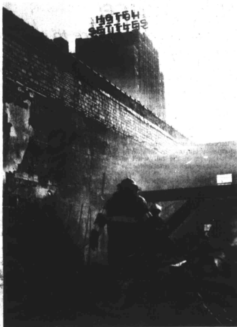
DOWNTOWN STORE DESTROYED — Big Spring firemen check for remaining small fires in what remains of Hudson Furniture Store at 315 Main. The store was destroyed by a fire that began late Wednesday night. The two-story building formerly housed J.C. Penney's department store.
