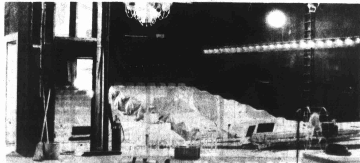
VIEW FROM THE STAGE — The 160 red seats of the opera house are covered with plastic for protection, but will be filled when the opera house reopens in
