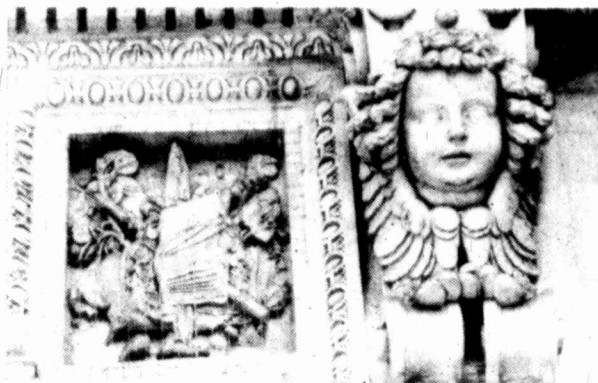
ANTI-PIGEON DEVICE — Electric wires adorn the artworks on the Milan Gothic Cathedral. The wires were installed to prevent pigeons from landing on the church's spires and statues which have been badly damaged by the birds.
