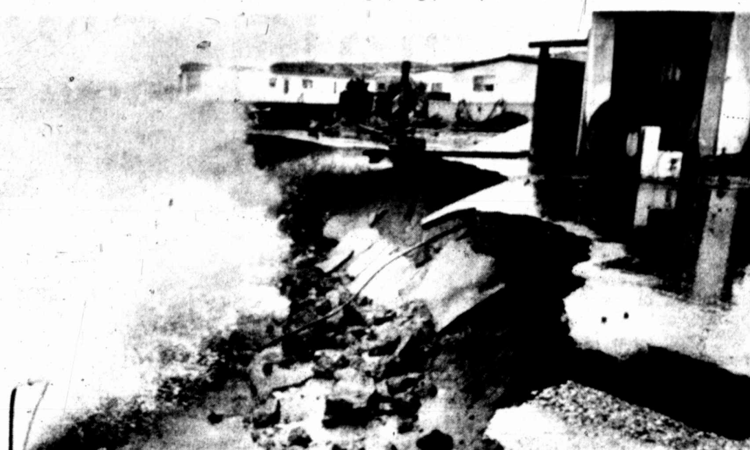
POUNGING SURF — The pounding Pacific Ocean tides are eroding the coastline at Pacifica, south of San Francisco, forcing evacuation of part of the Pacific Skies Estates trailer park.
