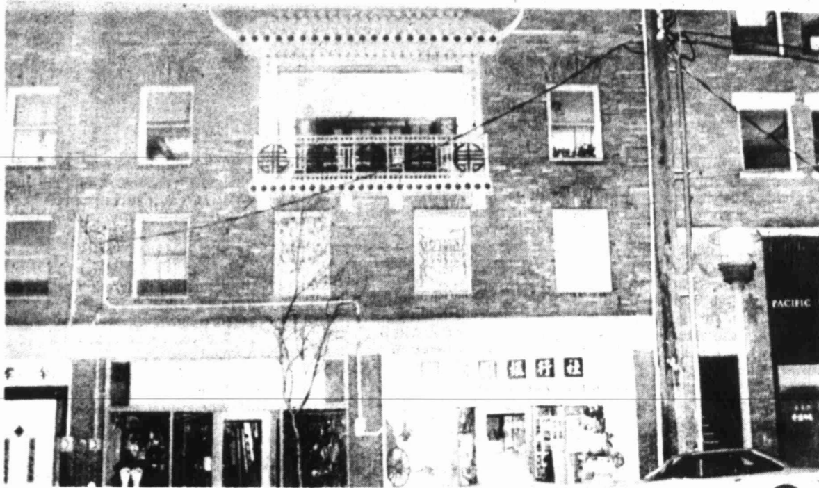
CHINATOWN — Police found 13 people dead behind these buildings in Seattle's usually quiet Chinatown area
