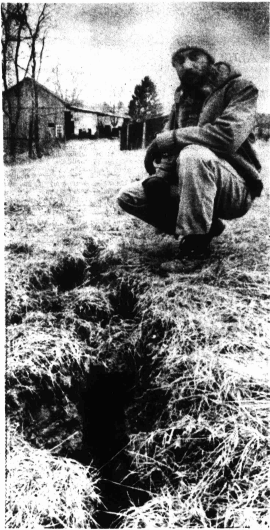
A CRACK IN THE LAND — Mark Spezza kneels next to a crack in the hill behind his Wilkesville, Ohio barn. Spezza believes the crack was caused by longwall mining of coal beneath his 57-acre tract. The cracks run through his century-old barn in the background.
