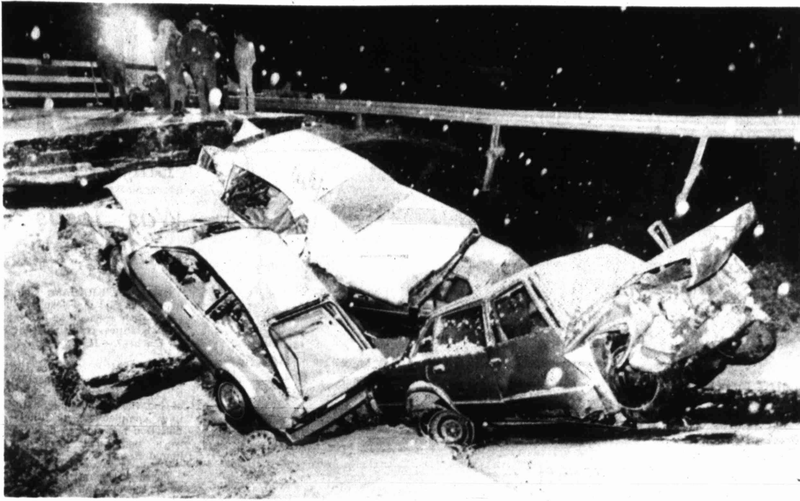
WRECKAGE — The twisted wreckage of four cars stacked one on top of another lies at the bottom of a culvert after a bridge on a county road collapsed Sunday near Antwerp, Ohio. Five people died and four, including a six-week-old baby, were injured.
