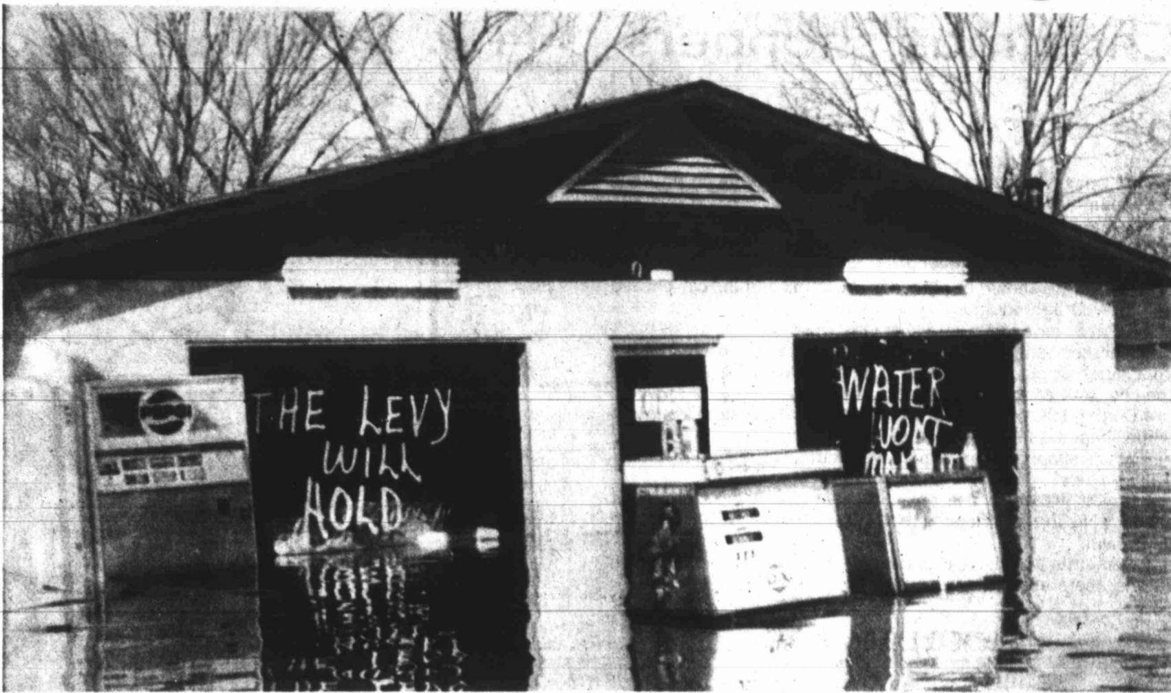
WRONG — A Jacksonport, Ark. store and service station owner wrote "The levy will hold" on the window of the business, but the levee obviously did not hold. Flood waters covered the entire town, and many parts of the Midwest braced for more.
