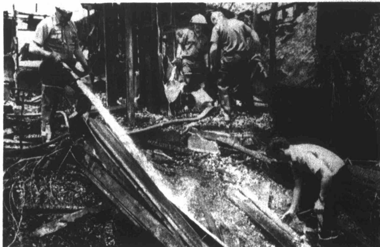
SIFTING THROUGH THE RUBBLE — Fort Worth firemen sift through the debris left after a fire burned a house near Lake Worth Sunday morning. The unoccupied frame house is the scene where four people were slain earlier this month. Fire officials have not ruled out arson.
