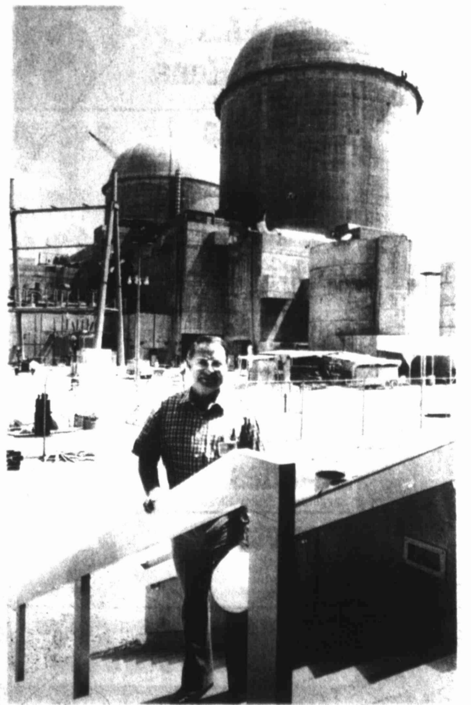
BIG SPRINGER — Hooper Sanders, a representative from the Big Spring branch of Texas Electric Service Company, pauses in front of the Comanche Peak nuclear reactor near Glen Rose. Sanders was part of a group of Big Spring TESCO representatives and media representatives which was recently treated to a tour of the plant. Texas Electric will be receiving a portion of the electricity produced here.
