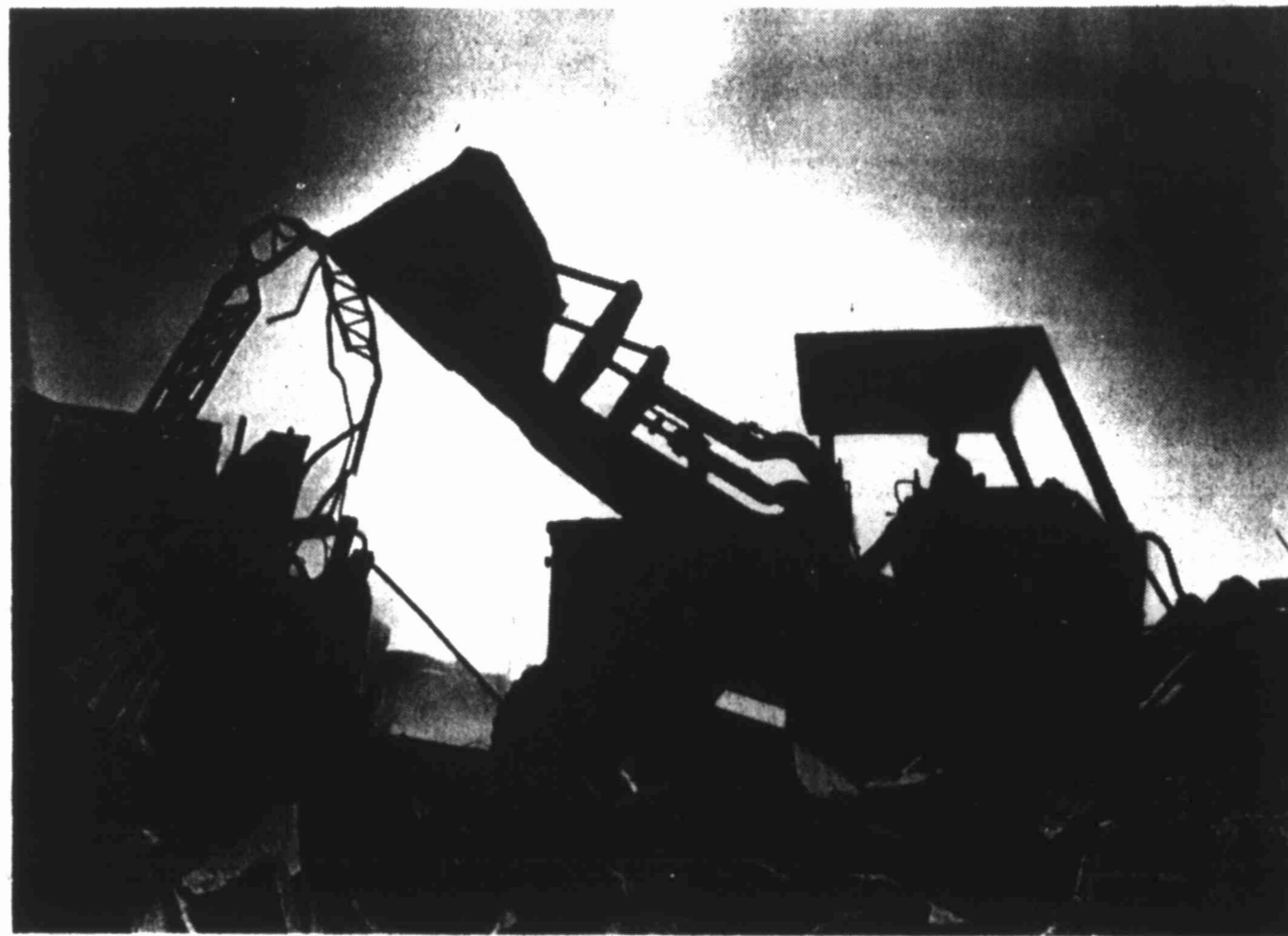
MUNCH A BUNCH — Another building bites the dust for progress as a bulldozer munches away at the Sheraton Motel in downtown Midland. The motel was sold to a local developer to build a new 37-story office building. The skyline of Midland is reaching higher as city planners approve more taller buildings.
