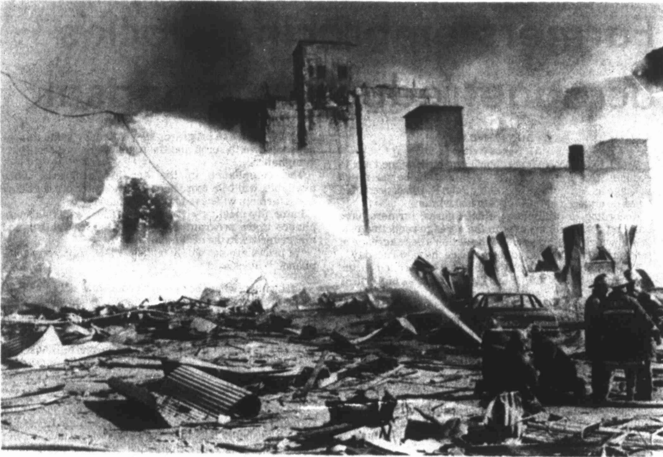
ELEVATOR BLAST —Firefighters pour water on a fire at a Council Bluffs, Iowa grain elevator Tuesday afternoon. The blaze broke out after an explosion at the elevator earlier in the afternoon. Twenty-two persons were sent to area hospitals with injuries.
