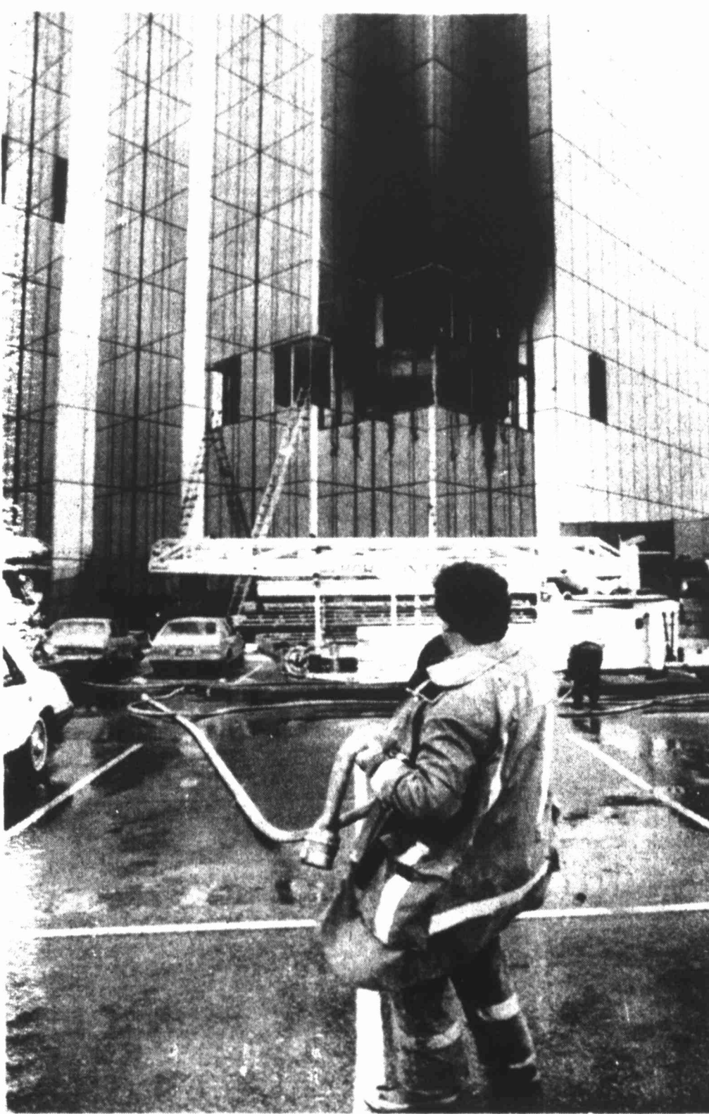
FATAL FIRE — A Houston fireman begins cleanup operations at the Westchase Hilton Hotel Saturday in Houston. A four-alarm fire killed 10 people and injured 11.
