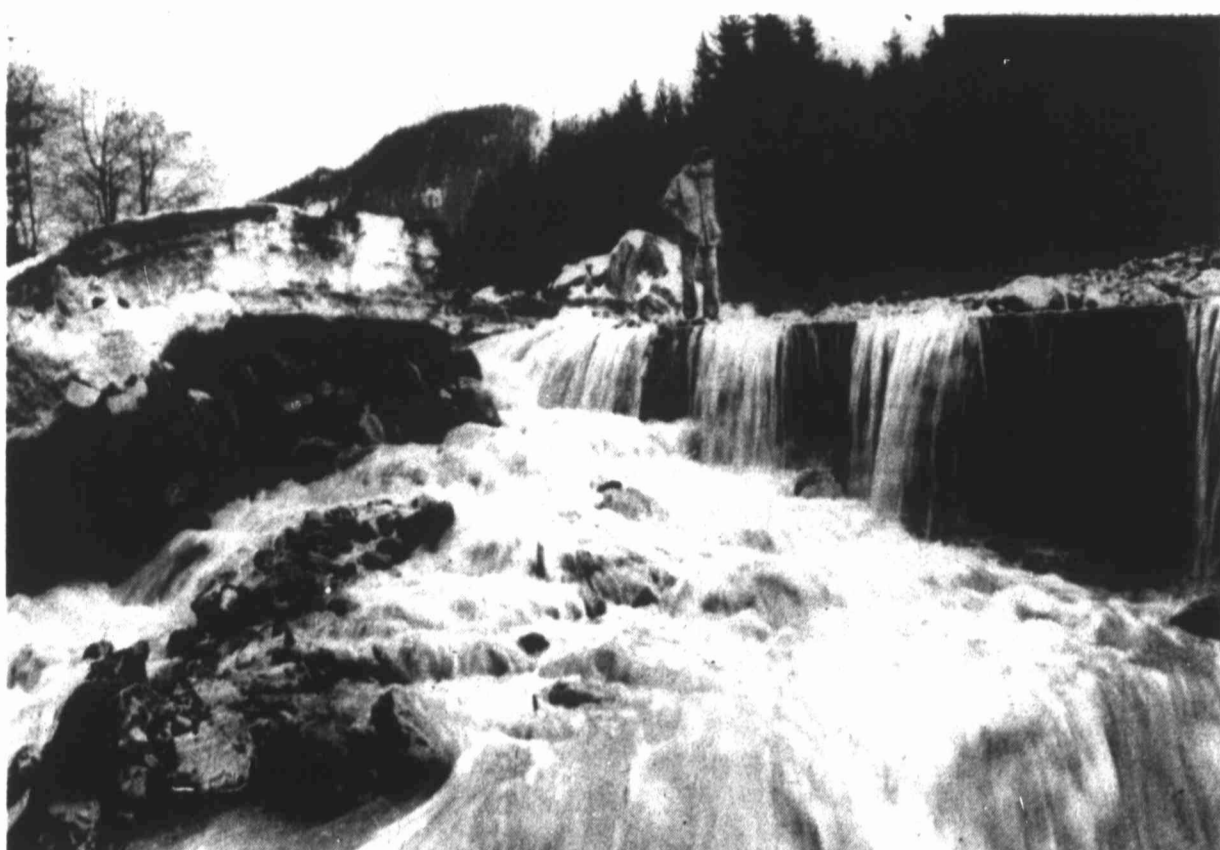
WATERFALL OVER HIGHWAY — An observer stands on an undermined portion of Interstate 90s eastbound lanes where rampaging Olallie Creek dumped tons of rock and dirt, then washed out portions of the highway's shoulder about three miles west of the Snoqualmie Pass summit. Cleanup and repairs on the damaged area of Washington's major east-west highway will take at least a week.
