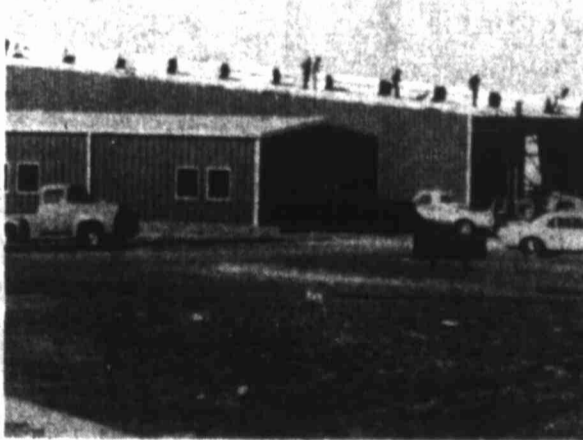
THE FIBERFLEX PLANT IN BIG SPRING...some of Chaparral Contractors' work
