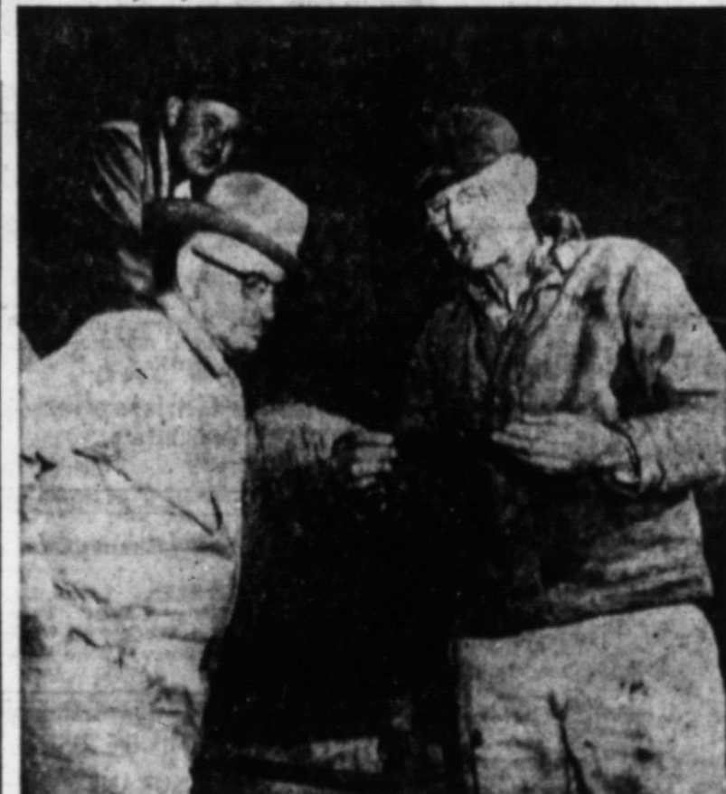
HOT ENOUGH? —Willie R. Stewart, top, and Earl Anthony, left, senior maintenance foreman for the Texas Highway Department here, watch as John Clark of 713 North Third, checks the temperature of hot tarring used to repair county highways. The material must be about 160 degrees before it can be used. (NEWSfoto)
