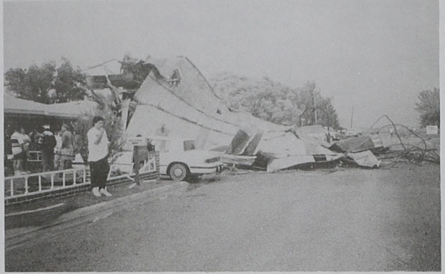
ROOF DAMAGE --The roof of the Stanberry garage ended up in the front yard and street in front of the Ureste home on Walnut Street. The metal roof did quite a bit of damage to the Ureste's house and yard.
