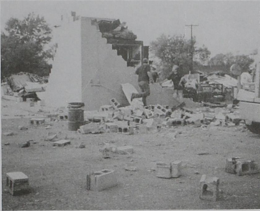
MECHANIC SHOP --The Stanberry Mechanic Shop at the corner of Highway 60 and Virginia Street was completely demolished, with concrete blocks from the building scattered all over the Drake Addition.
