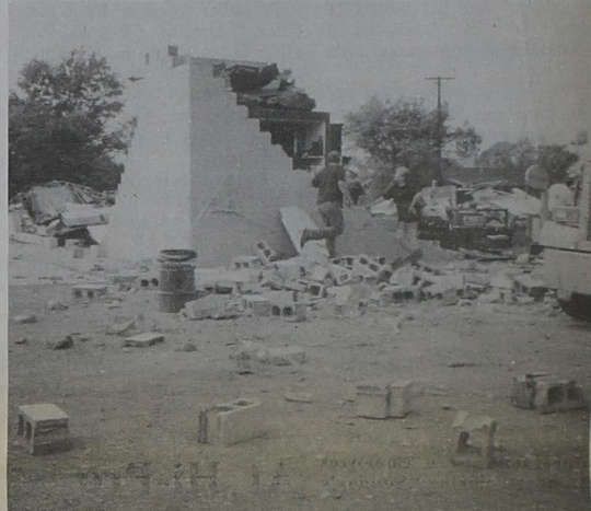
MECHANIC SHOP --The Stanberry Mechanic Shop at the corner of Highway 60 and Virginia Street was completely demolished, with concrete blocks from the building scattered all over the Drake Addition.
