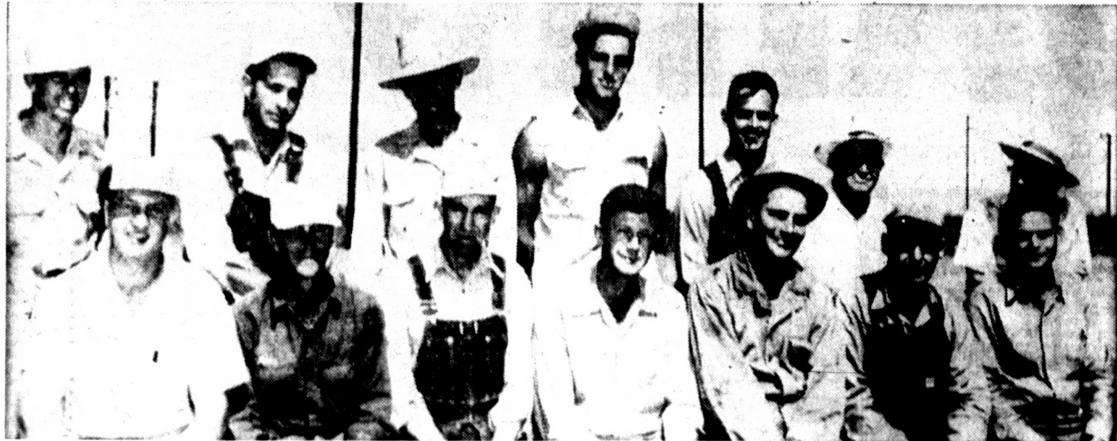
OZARK-MAHONING EMPLOYEES —Construction is well under way at Ozark-Mahoning company's plant site 14 miles east of Brownfield. Employees took time this week for the picture above. From left in front, they are Bruce Anderson, Perry Stokes, L. T. Brinson, Bob Cummings, Walter Selcer, Elton Young and Jim Hogan. From left and standing: Drew Hobdy, Bryce Wagoner, Tommy Shipman, Milfred Ratliff, Ed Lofton, R. R. Marsh and Bill Coghill. Coghill is of the company's Tulsa offices, and Marsh is plant superintendent here. (Staff Photo)
