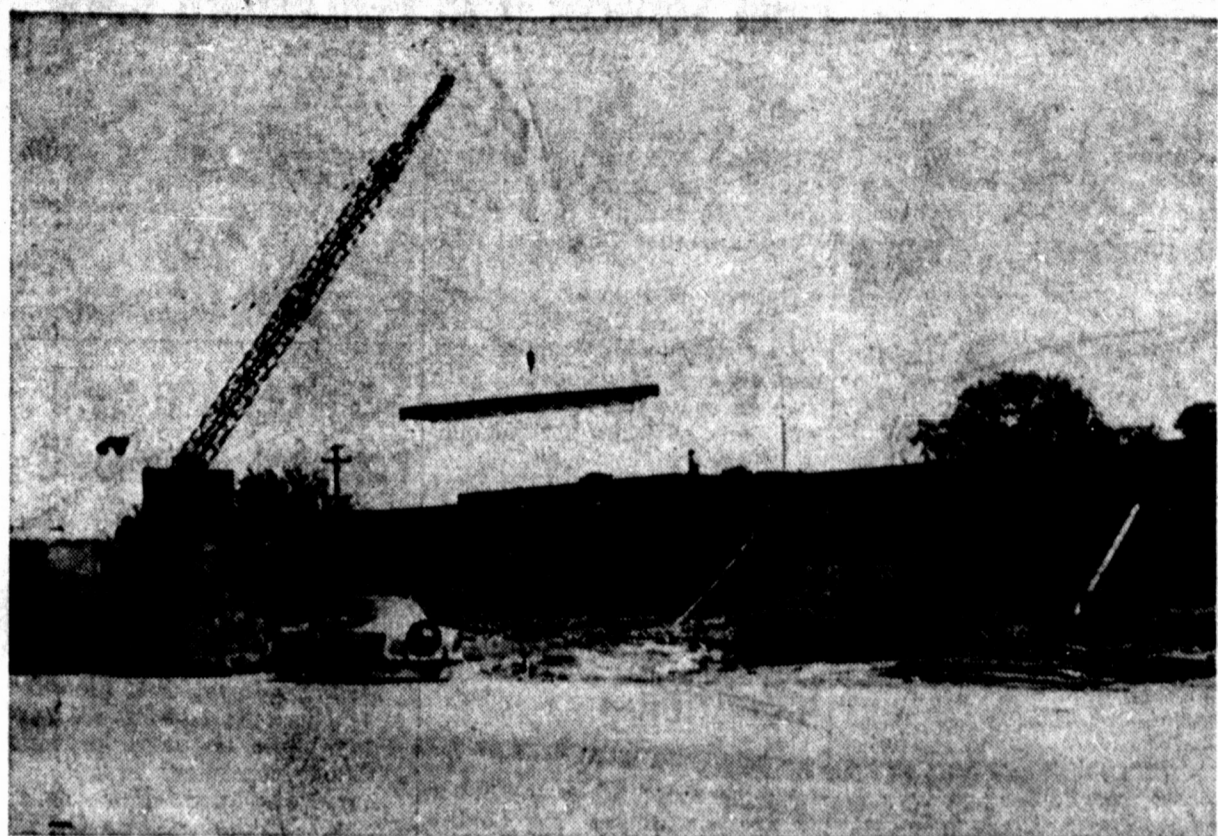
NEW CONSTRUCTION —The future home of Lindsey's Hardware fast is taking shape at Broadway and Lubbock road intersection. To contain 84,000 square feet, the building—of steel and concrete—will be enhanced by a 150-foot pane of tinted glass in the front—facing west. Roger Lindsey said this morning that he expects to occupy the building about Sept. 1. In the picture above, steel beams are being swung into place for the roofing system. When completed, the building will be the largest retail store in Brownfield in point of floor space. (Staff Photo)
