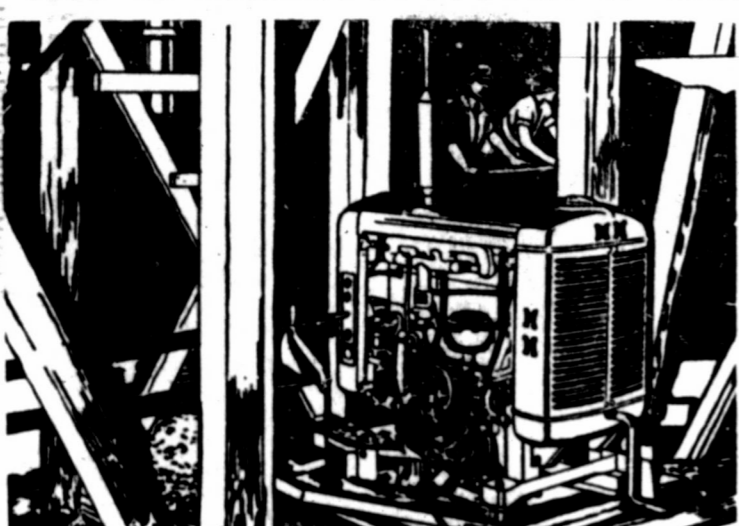
MM 403-4A Power Unit Supplying Lumber Mill Power
