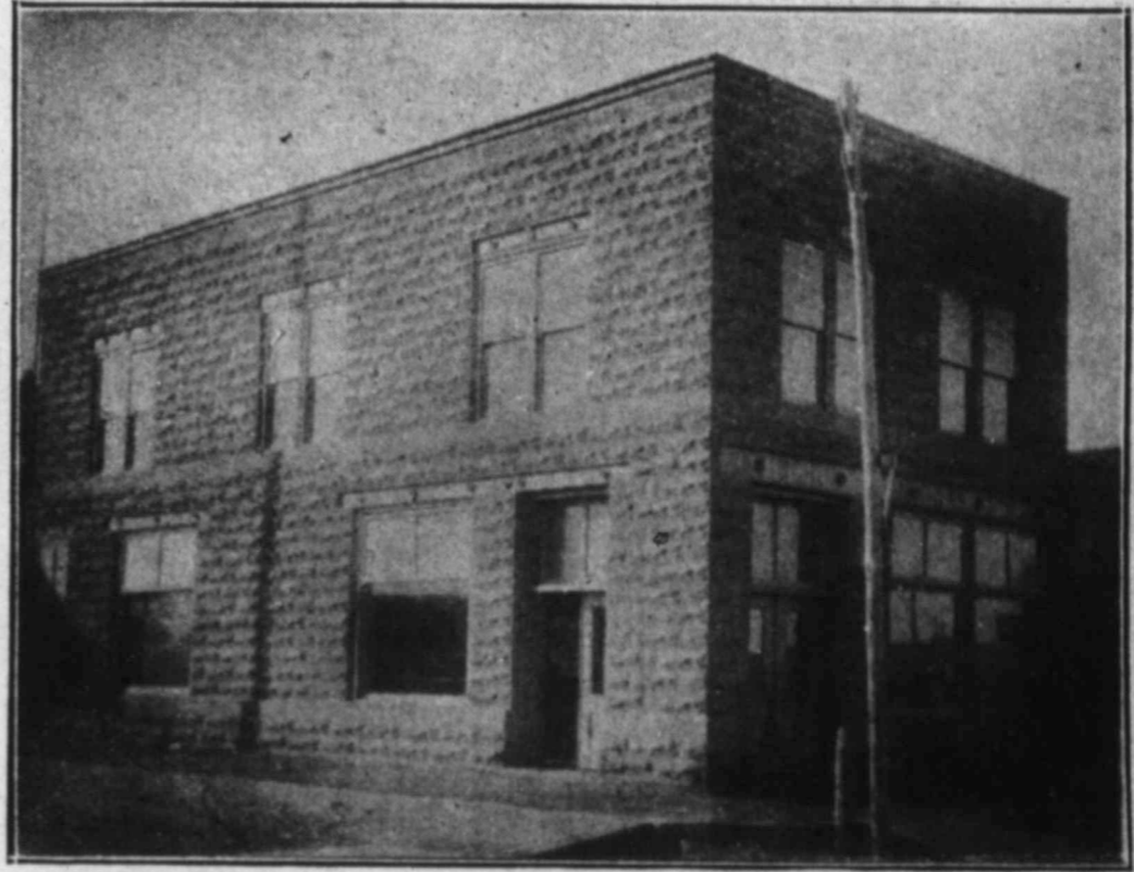
U. S. POST OFFICE BUILDING, WOODWARD.
