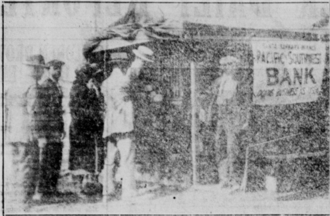
Earthquakes don't worry this bank! The Santa Barbara branch of the Pacific Southwest bank found its regular quarters all in a heap, so officials erected a tent and conducted business as usual. It was the first bank to open after the quake.
