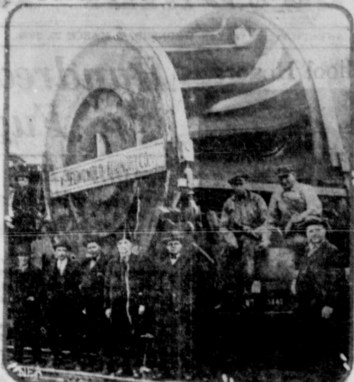
This turbine casing, 17 feet high weighing 70 tons is to become part of the gigantic power plant at Wilson Dam, Muscle Shoals. From the foundry at Wheeling, W. Va., to its destination the route was carefully calculated and tunnels measured to avoid those that were too small.
