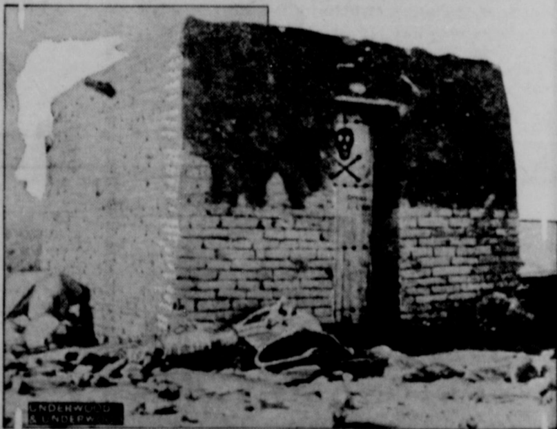
Here is the oldest railroad station in the world, insofar as the material used in its construction is concerned. The station, built almost entirely of bricks which date to the reign of King Ashurnasirpal, over 3,500 years ago, has just been erected on the Khorsabad railroad at Tell Billa in Mesopotamia by an archeological expedition from the University of Pennsylvania museum and the American School of Oriental Research in Bagdad. It serves as a shipping depot and storage house.
